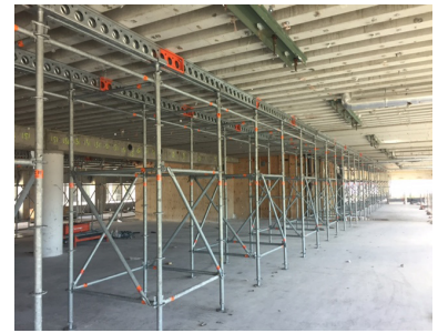
Back propping for demolition
