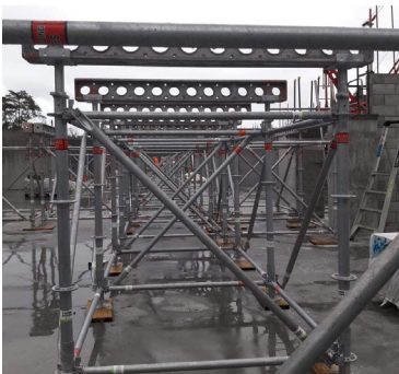
Midspan and beam propping in commercial construction
