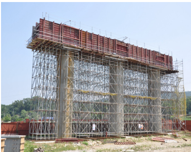
Heavy duty civil construction
